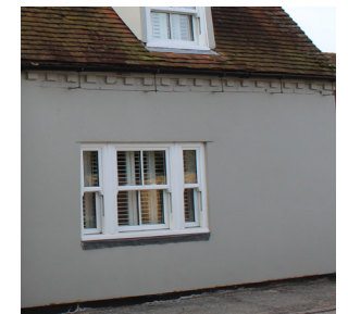
Figure 24 Example of the use of render with timber windows and a plain tile roof
