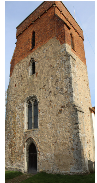
Figure 19 The tower of St Lawrence Church
