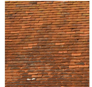
Figure 22 Example of Red Plain Clay Tiles
