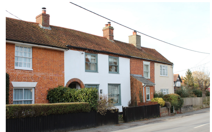
Figure 43 The group value of terraces is particularly vulnerable to incremental change
