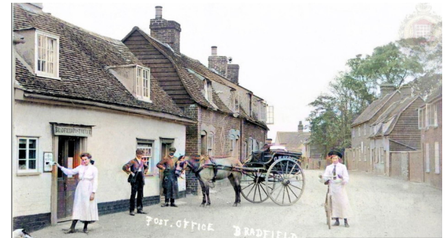
Figure 14 The Post Office, now demolished ©Nigel Klammer
