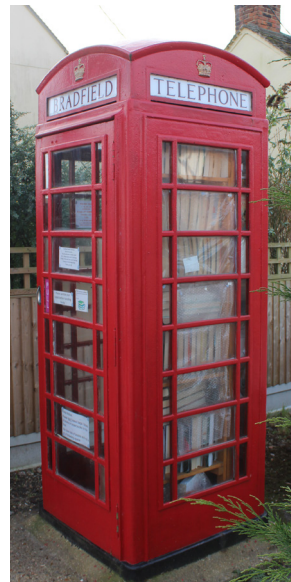
Figure 34 Listed K6 Telephone Box
