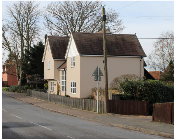
Figure 3 Old Hall House, which has been removed from the Conservation Area
