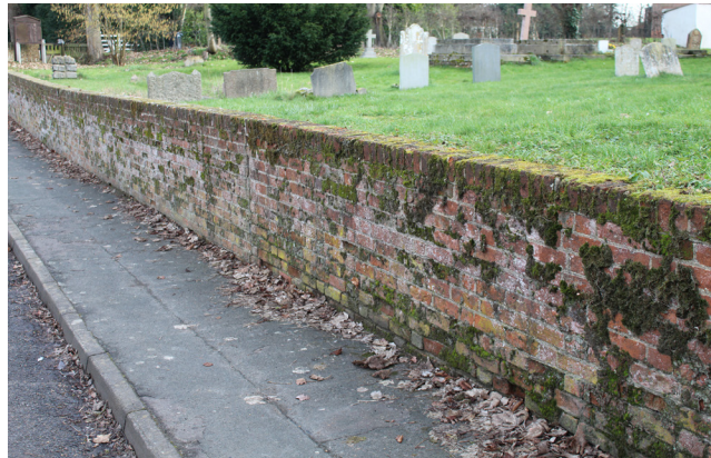
Figure 44 The boundary wall to the Churchyard is in need of maintenance and repair
