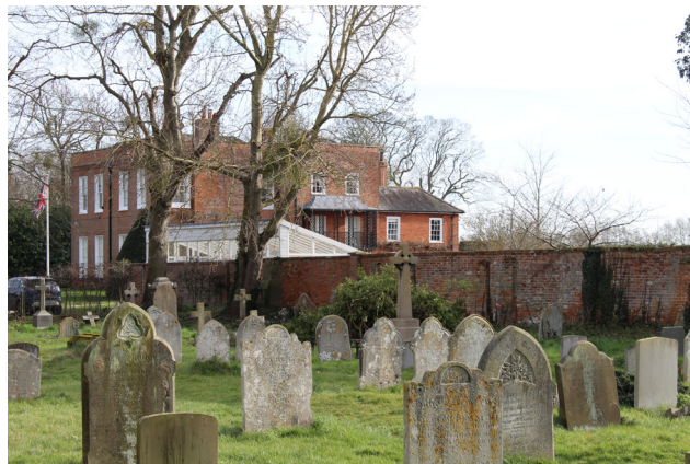
Figure 32 View towards Bradfield Place from the churchyard
